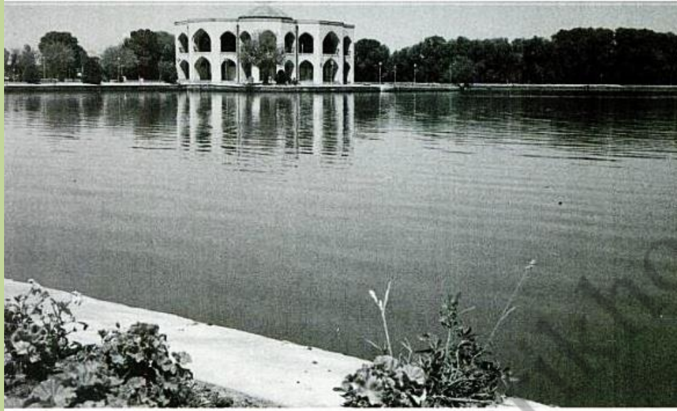
153 The octagonal pavilion – perhaps once crowned by a dome – set in the large artificial lake, or Royal Pond, at Tabriz. Viewed from the adjacent hill, the water seems to hover over the surrounding valley.
